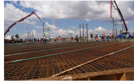
The first time a pre-tensioned floor had been used for a reservoir in Africa
