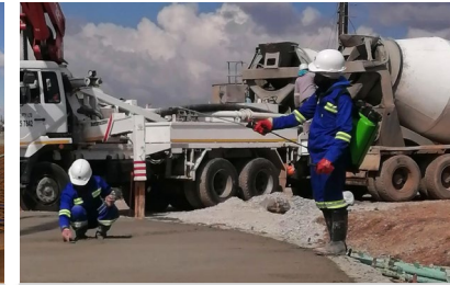
Evaporation controlled with CHRYSO® Profilm 19 evaporation reducer
