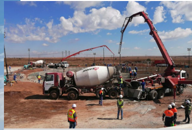
212 truckloads of concrete poured from 3 nearby batch plants in one day
