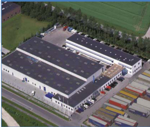
BWT HOH, Greve, in Denmark
