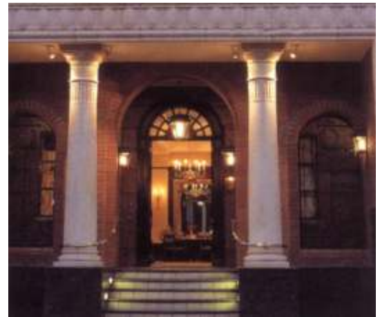
In-Situ cast columns supplied and installed by Old World Concretes (Pty) Ltd.
