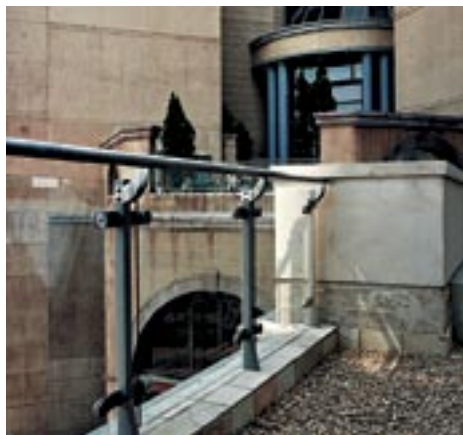
Michelangelo Towers, Sandton Architect: Bentel Associates International Product: 10 mm clear Armourplate
