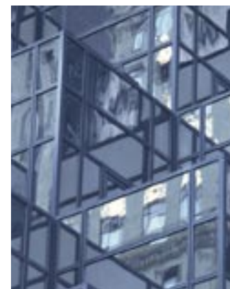
Activ™ self-cleaning glass reduces maintenance costs and the risk of damage during cleaning.
