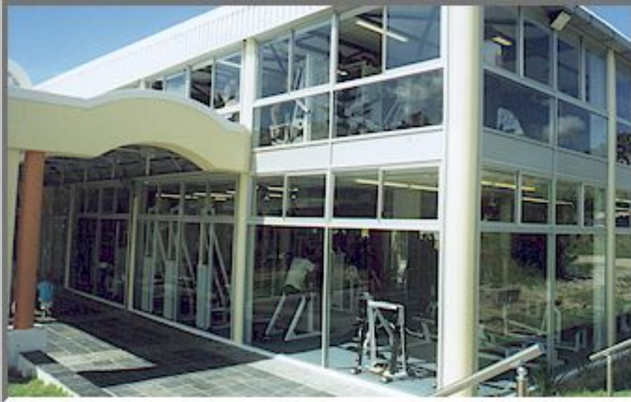
Health and Racquet Club - Constantia Manufacture and installation of curtain wall units
