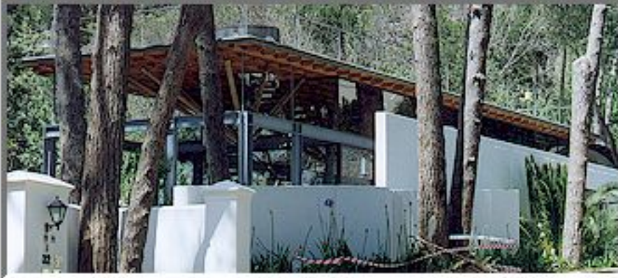
The Tree House, Oranjezicht Manufacture and installation of doors and windows.
