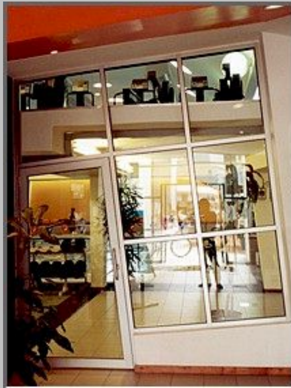
H&RC - Claremont, Cape Town Foyer door.
