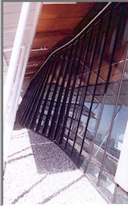
Seafisheries Restaurant - Sea Point Manufacture and installation of curtain wall
