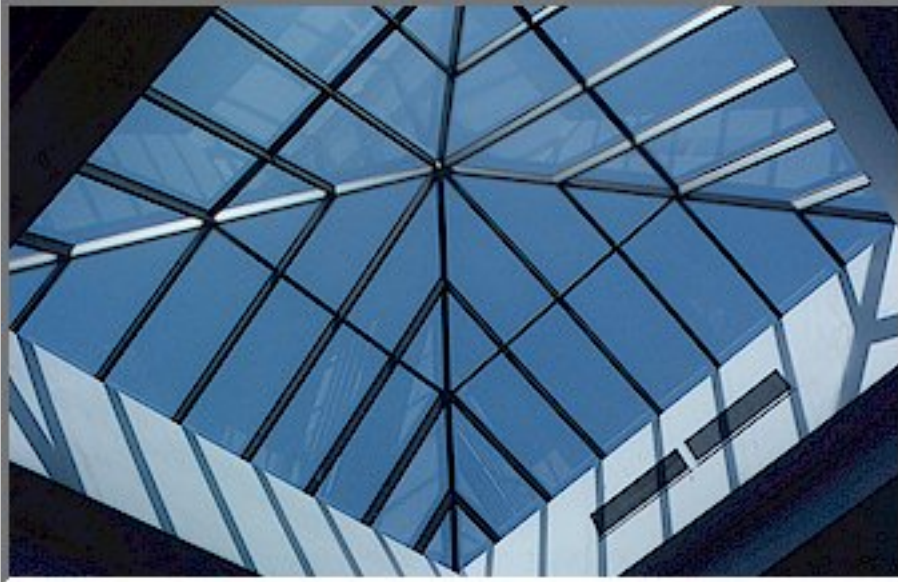
Christian Network Building - Bellville Manufacture and installation of skylight.
