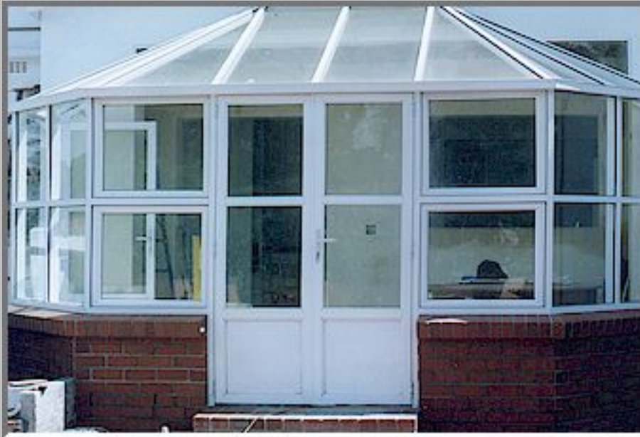
Private Residence - Rondebosch Manufacture and installation of conservatory.
