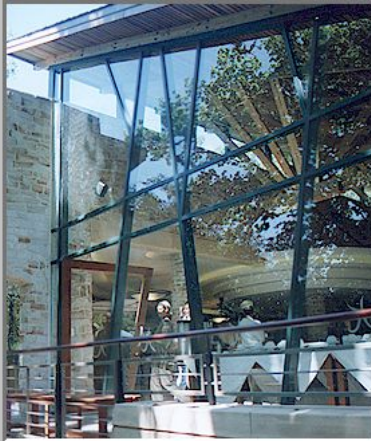
Kirstenbosch Restaurant Manufacture and installation of curtain wall units.
