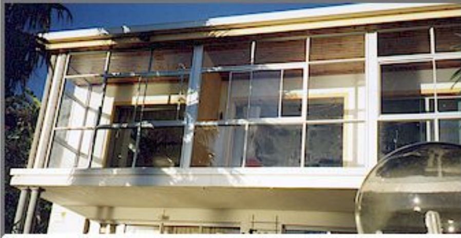
Private Residence - Camps Bay Manufacture and installation of balcony enclosure.
