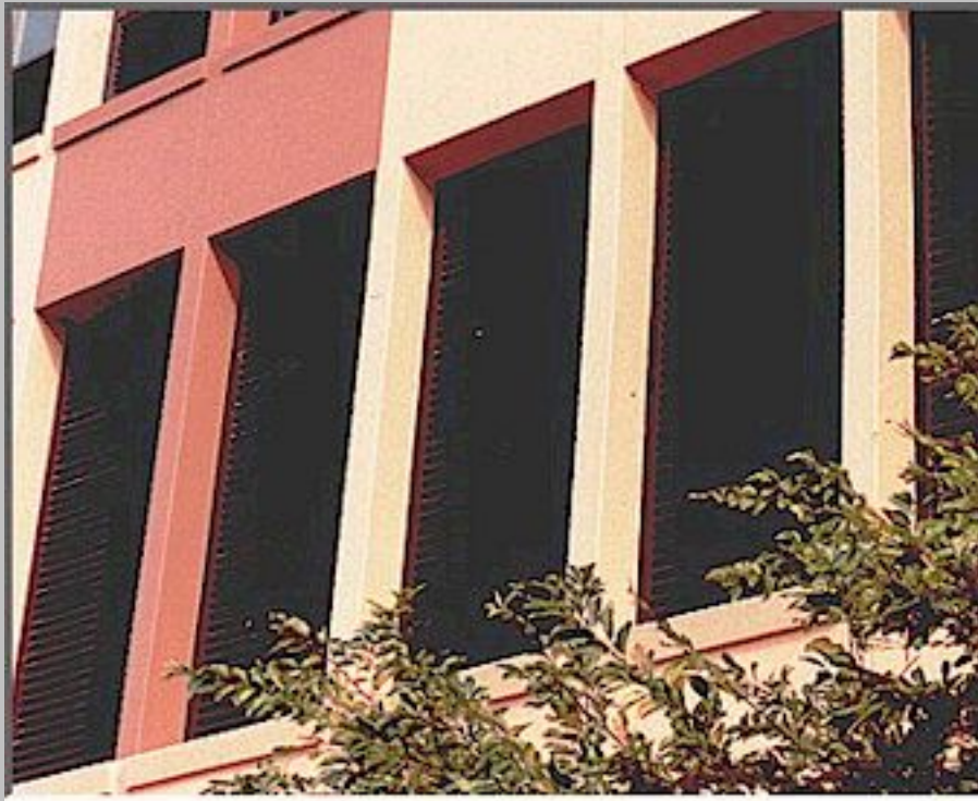
CCMA House - 78 Darling Street Manufacture and installation of aluminium louvres.
