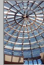
ALISSA SHOPPING CENTRE Al Khobar (Saudi Arabia) Design of aluminium and glass dome.
