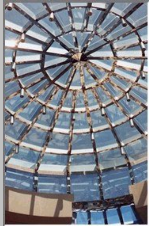
ALISSA SHOPPING CENTRE Al Khobar (Saudi Arabia) Design of aluminium and glass dome.
