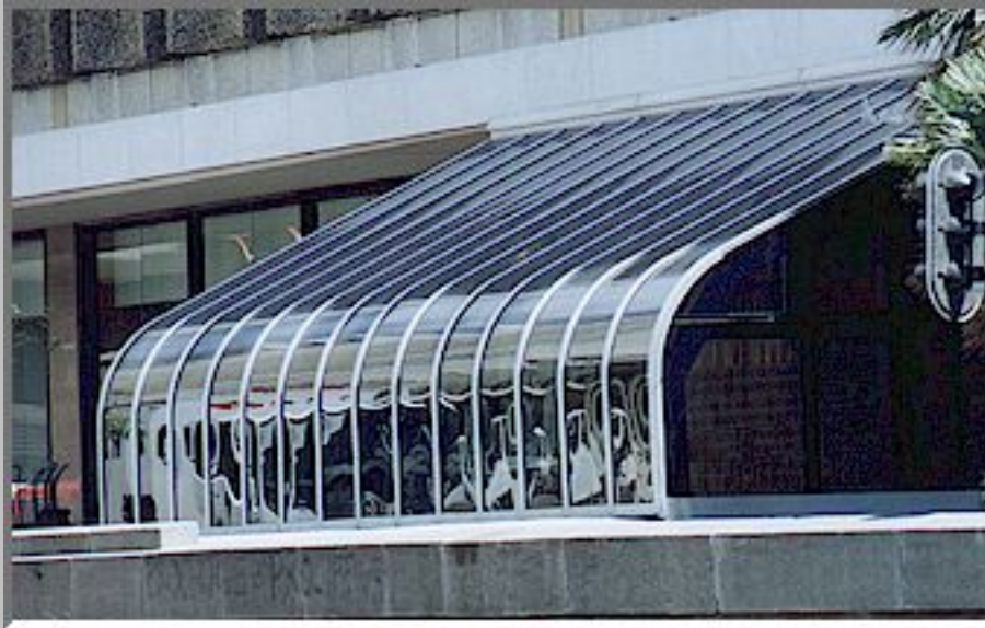
Strand Concourse - Adderley Street Cape Town Installation of escalator canopy.
