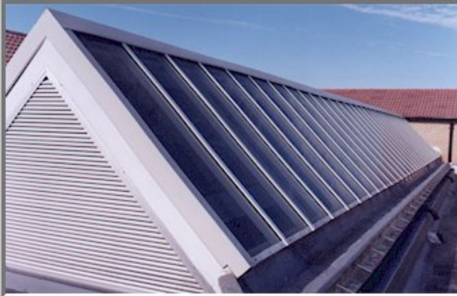
ABC Building, UWC - Bellville Manufacture and installation of skylights.
