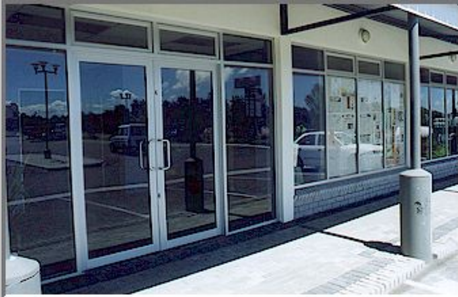
Bracken Manor - Brackenfell Manufacture and installation of shopfronts.
