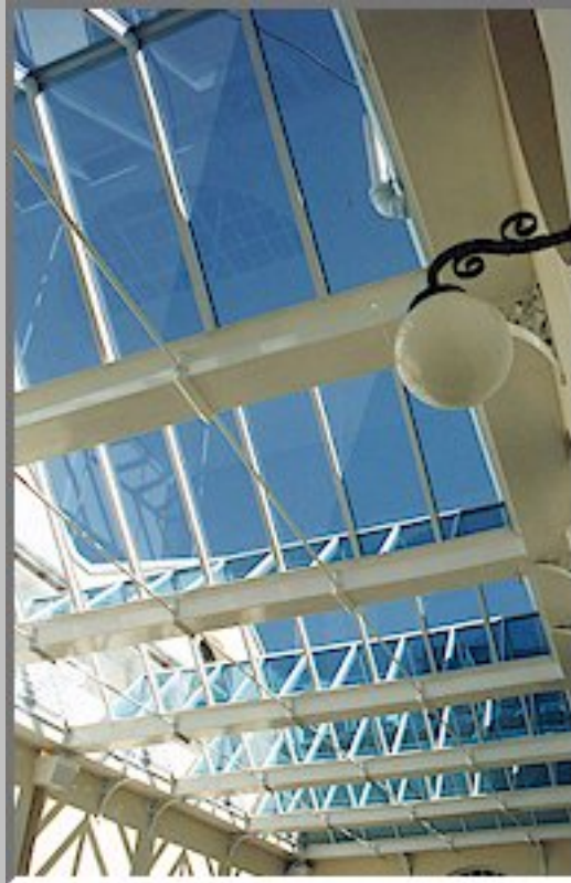
Supreme Court - Cape Town Manufacture and installation of skylights.
