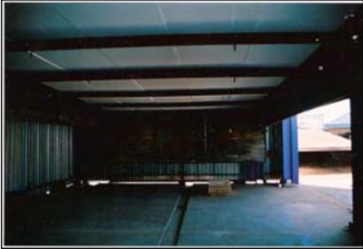
Figure B1-1: Installation prior to ignition of fire source
